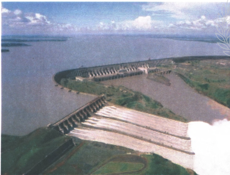
Fig.1. Total view of ITAIPU. Left part shows overflow (spillway).
