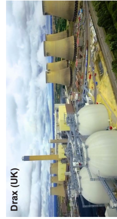
2,595 MW e in total, 100% biomass (wood pellets)
