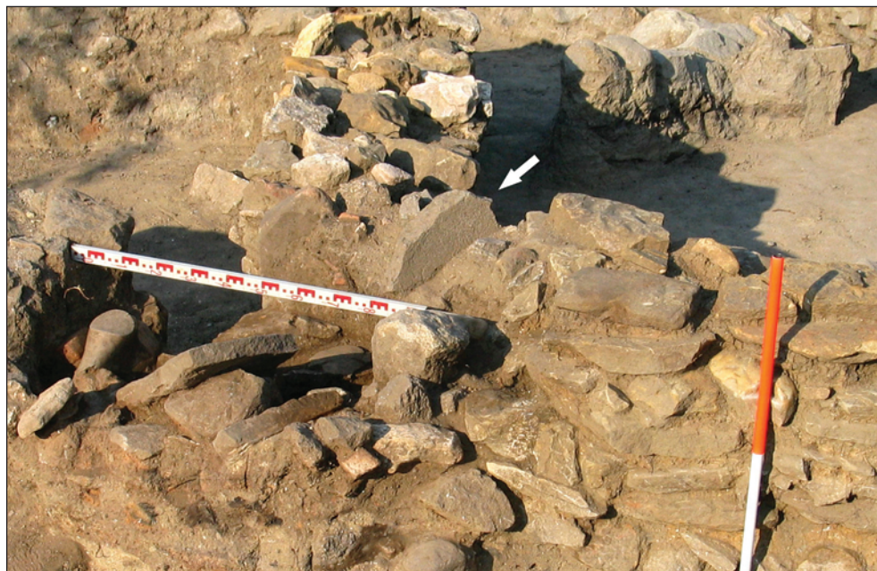
Fig. 2 Acropolis, fragment of millstone in the wall of northern building, 2003
