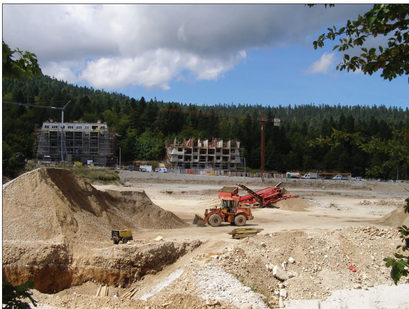
Slika 6. Gradnja novih objekata (oktobar 2023) Figure 6. Construction of new buildings (October 2023)
